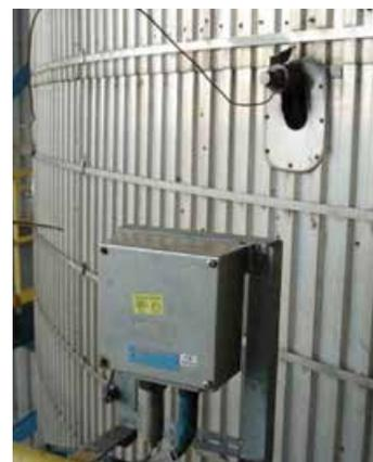
High-temperature accelerometers monitor vibrations on the coke drum wall. The resulting signals provide the operator with information regarding drum cleanliness status.
